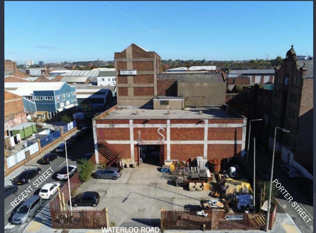
Existing Property Waterloo Road Elevation
